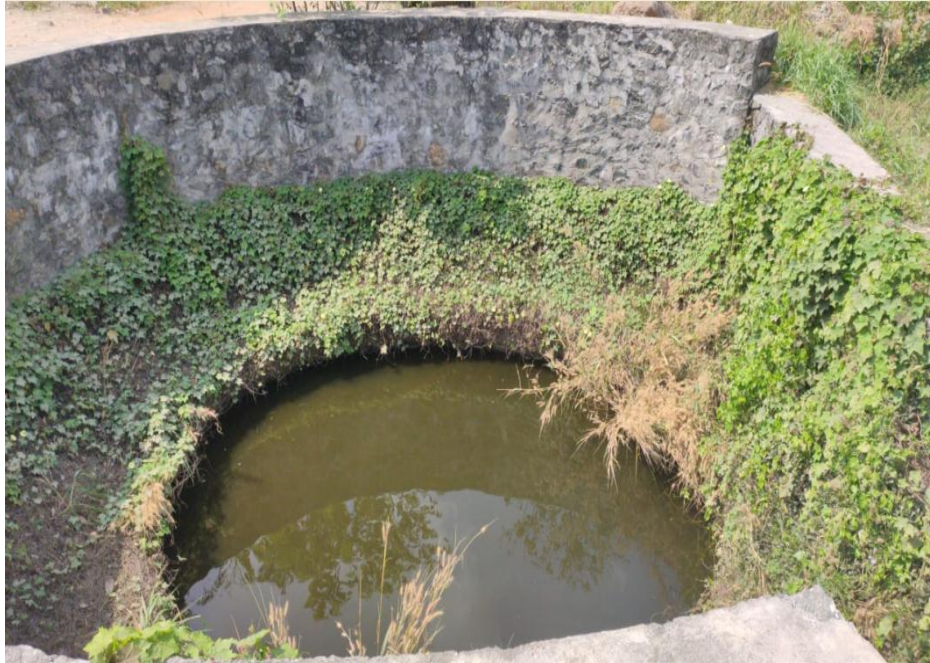
PLATE G: 1- Rainwater harvesting pits.
